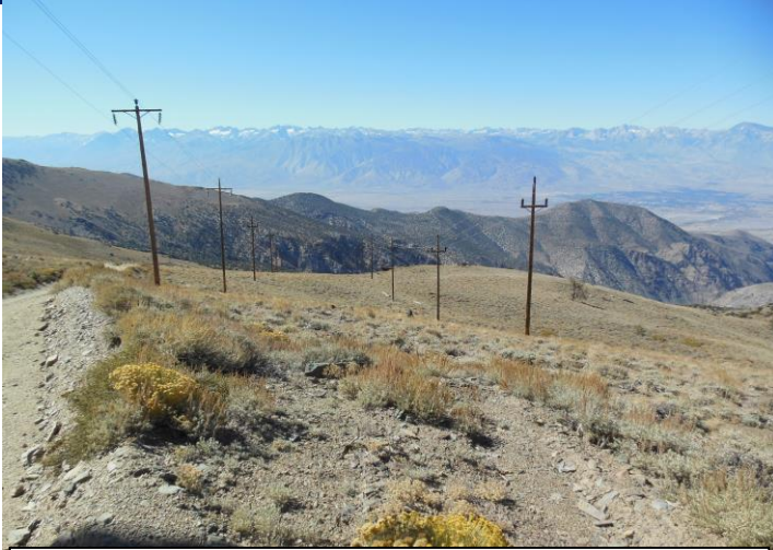
Existing subtransmission lines in Segment 3 going up Silver Canyon Road.
