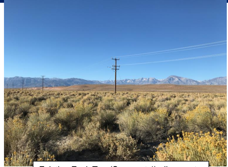
Existing Zack Tap (Segment 4) alignment.
